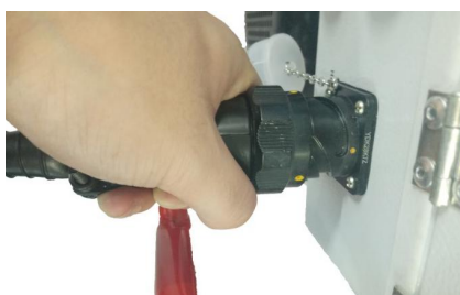
Connection the cable with electrical box
